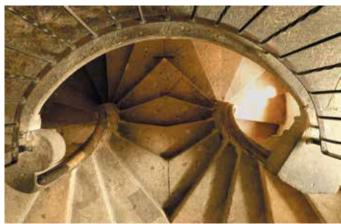
Fig. 8 Double spiral staircase
