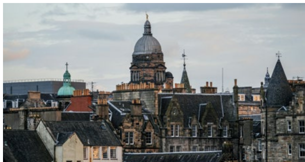
West Register House dome
